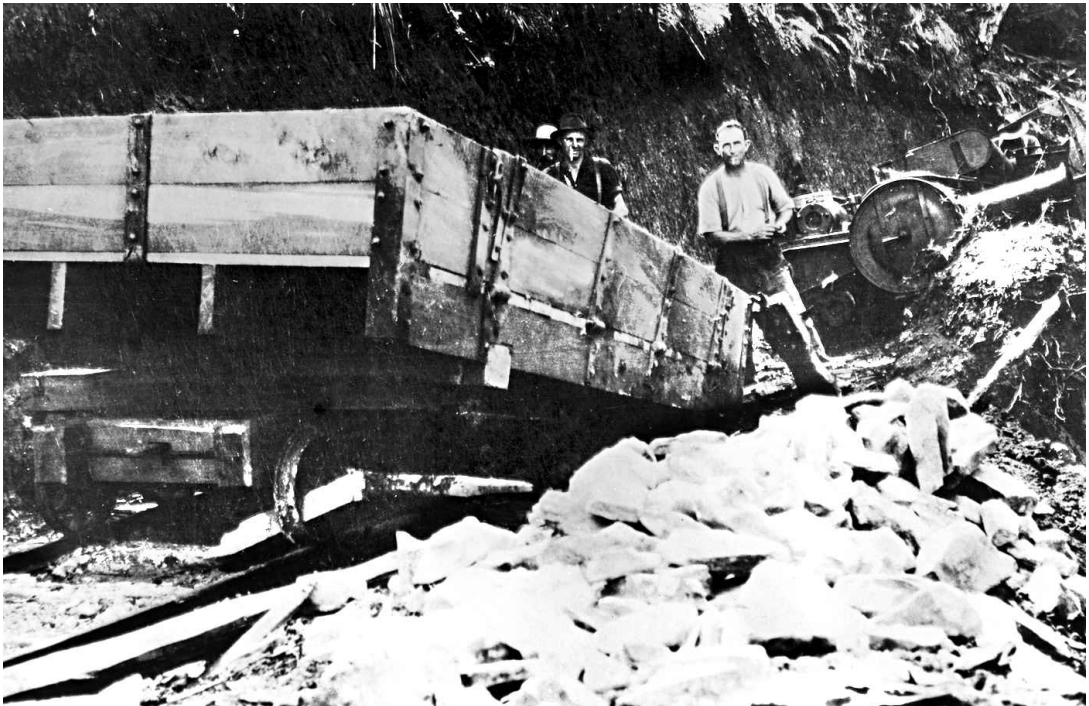
↑ A derailment on the quarry tramline. March 1928. ↓ Workers have unloaded the rocks from the wagon. 'There were some derailments in the first few weeks on the quarry line, until it settled into position, but on the whole, accidents were very few.' The man in the white shirt holds a timber jack, to push and lift the wagon into place.
