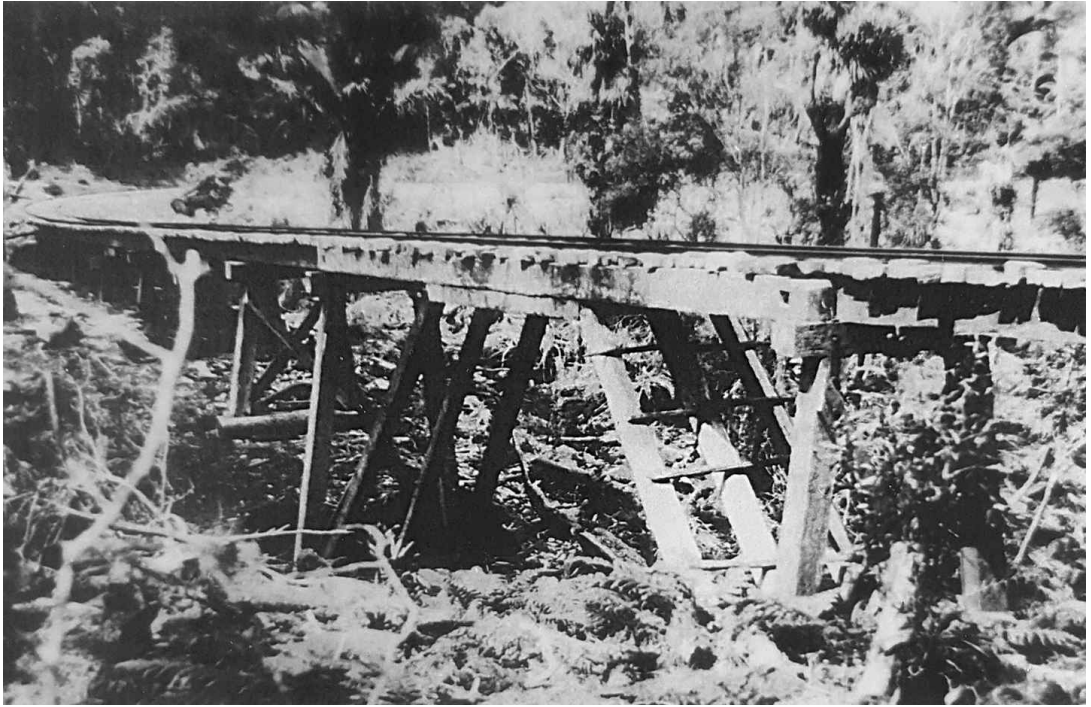
↑ Castles Bridge, looking down Huia Valley.
