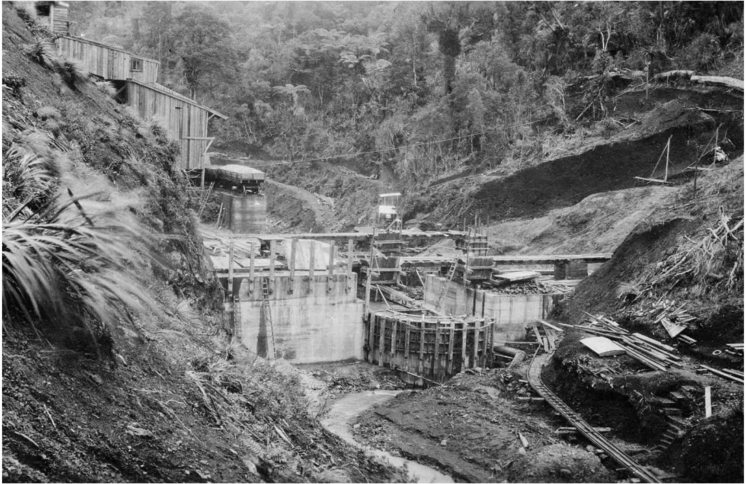
↑ Looking downstream to the dam. June 1928. The building is the crusher, with a wagon of sand beside it. The concrete mixer is under the crusher, to the left of and below the wagon.
