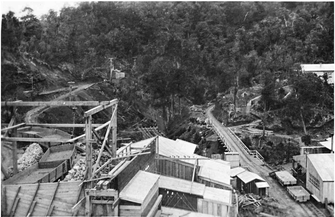
↑ Looking downstream to the dam. June 1928. The building is the crusher, with a wagon of sand beside it. The concrete mixer is under the crusher, to the left of and below the wagon.
