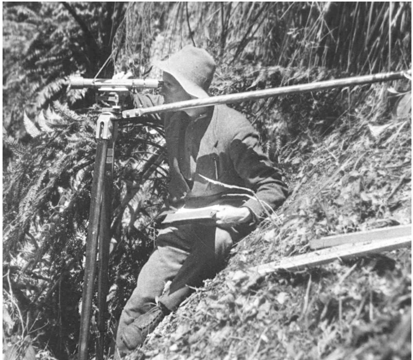
Arthur Mead surveying at the Huia dam site. He has had to extend a tripod leg back to steady it.
