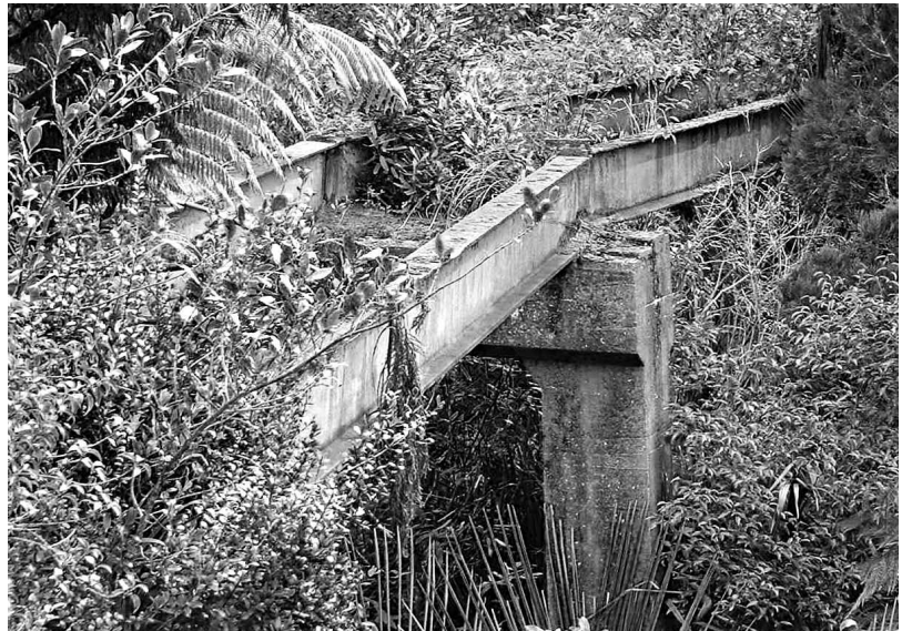
A bridge pier, 2004.
