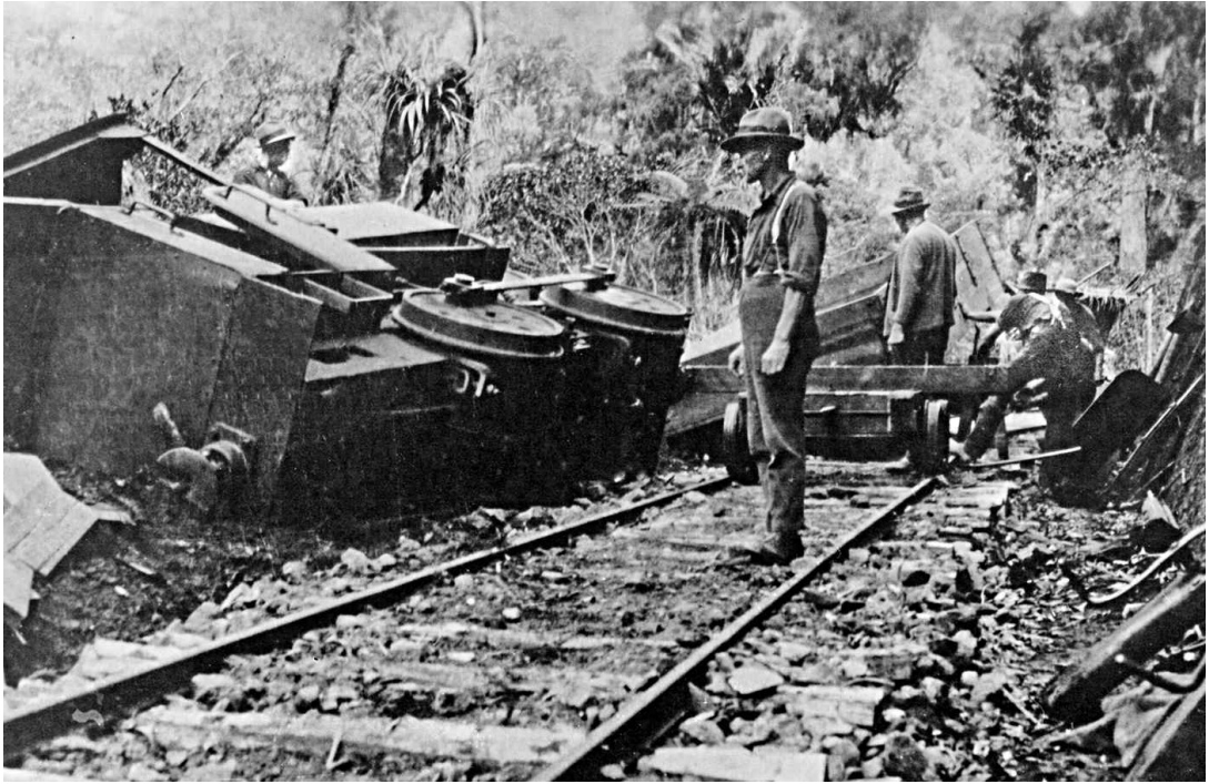
↑ A derailment on the quarry tramline. March 1928. ↓ Workers have unloaded the rocks from the wagon. 'There were some derailments in the first few weeks on the quarry line, until it settled into position, but on the whole, accidents were very few.' The man in the white shirt holds a timber jack, to push and lift the wagon into place.
