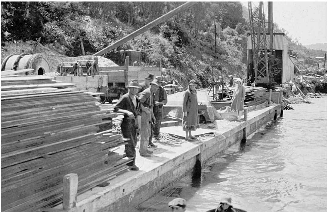
↓ Waiting for a launch. December 1929. The photo seems to have been taken from the launch's wheel-house roof — the bow is just visible. The dam is finished, the buildings have been demolished and supplies are being taken away.
