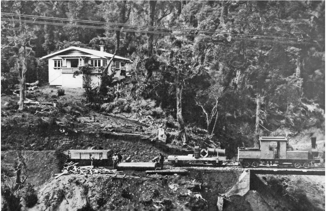
↑ The Price locomotive with water pipes, about 120 metres down from the dam. February 1928. The Price is on Huia Bridge. The new cottage is for the engineers, then the caretaker.
