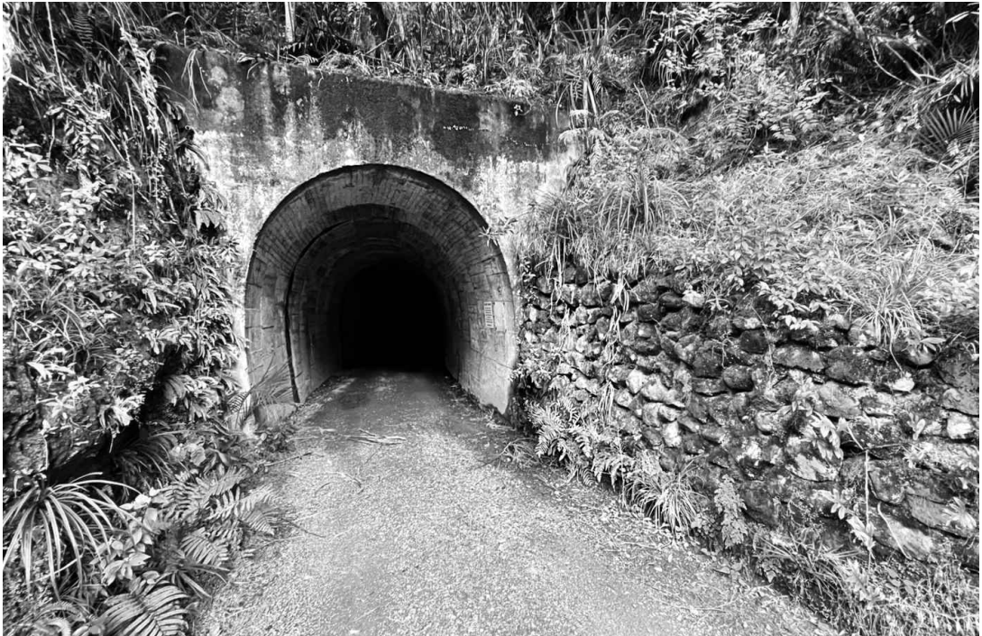
↓ The north end of the long tunnel, just up from Lincoln Bridge. This end originally had a timber roof to deflect falling rocks, but it was soon replaced with this concrete lining.
