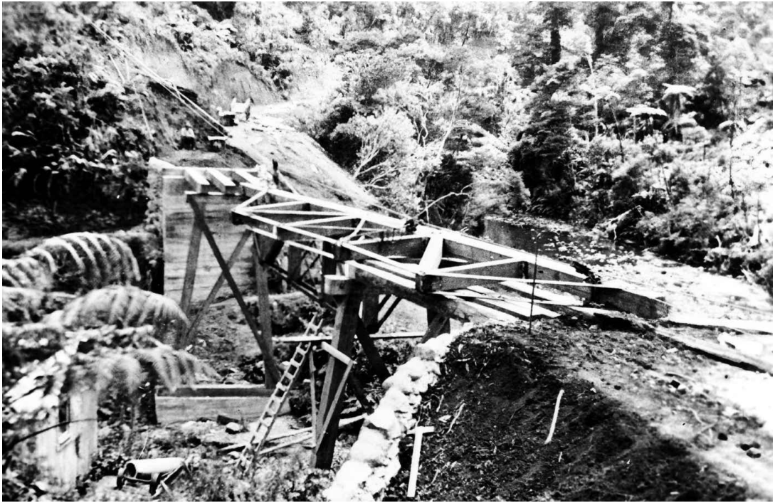
↑ Building Georges Bridge. Early 1926. One truss is in place and the second is being slid across.
